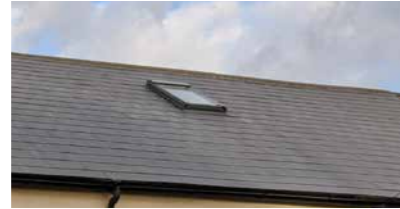
Grey slate roof tiles
