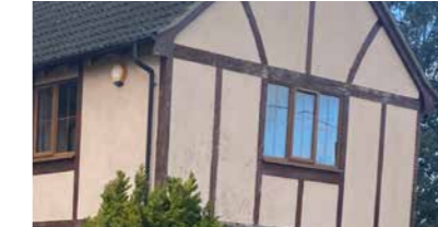
Timber framed (mock tudor)
