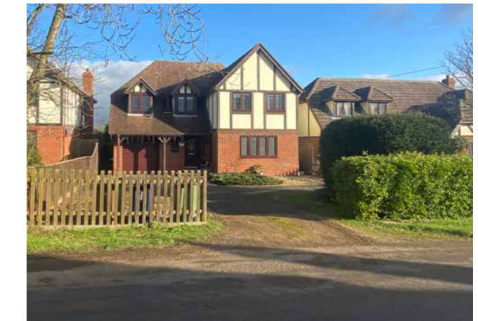
Figure 57: Local example of timber fencing and hedgerows being used as boundary treatment.
