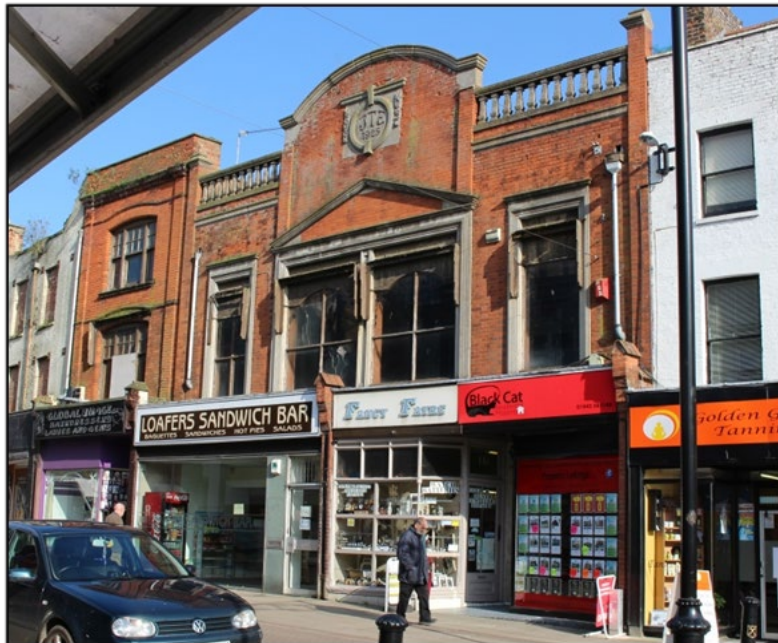
13-17 High Street – grant application approved for new shopfronts, first floor conversion and brickwork repair
