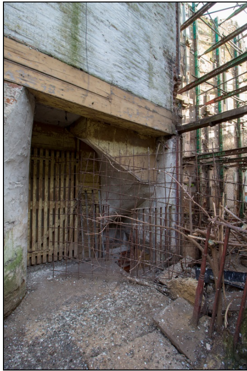
Elevation as viewed from the courtyard
