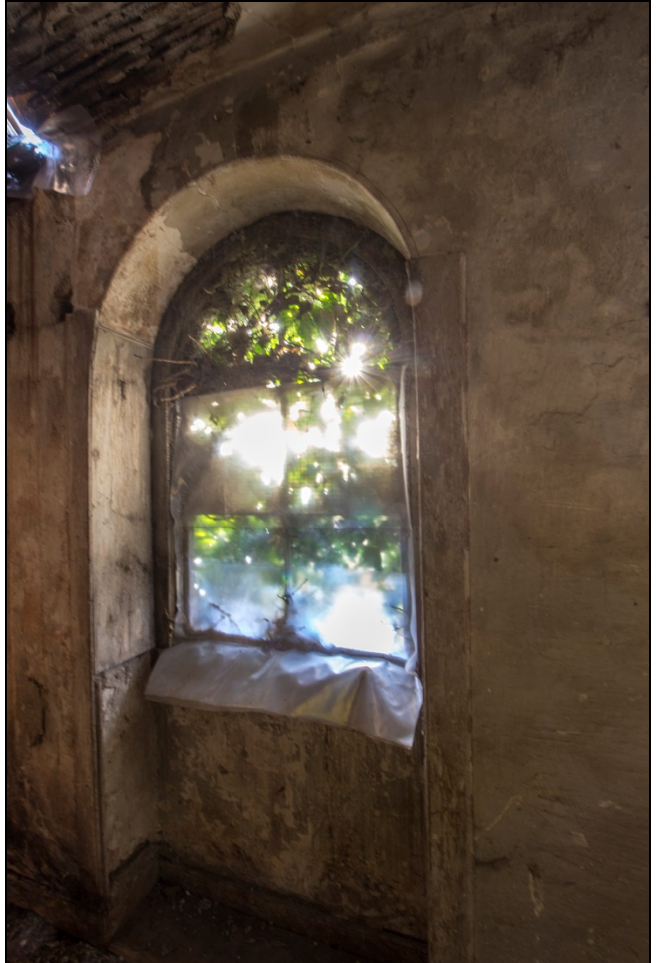
Second floor window
