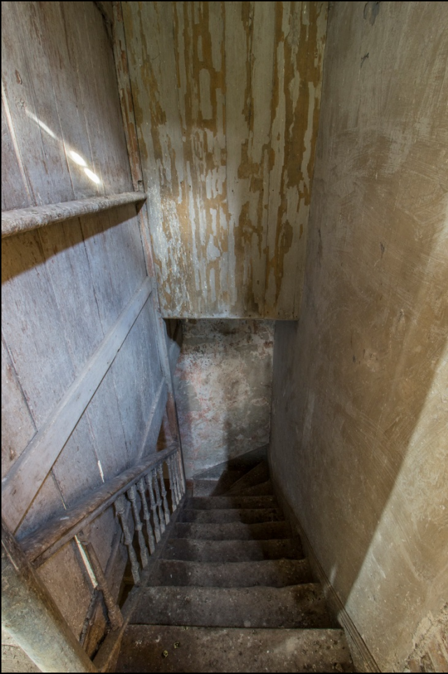
Looking down the stairs from first floor
