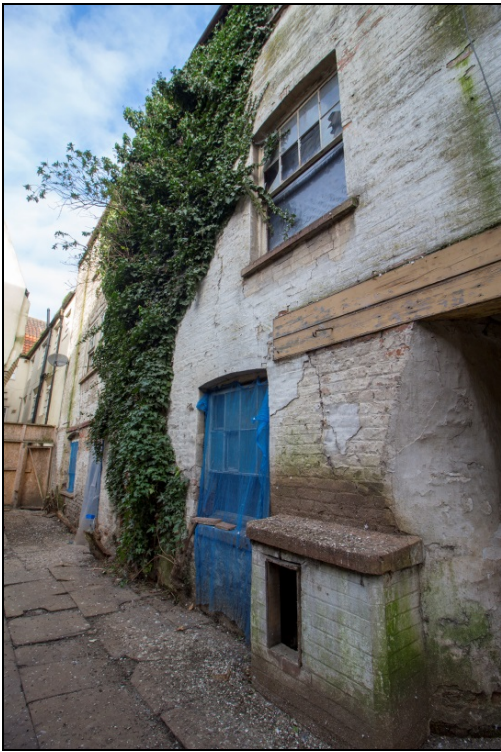
Elevation as viewed from the courtyard
