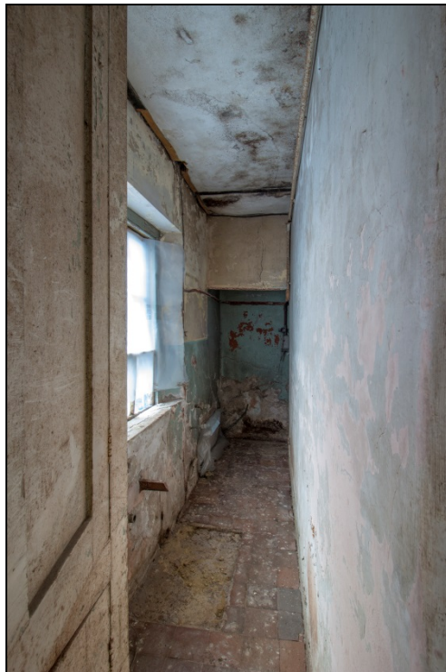
Ground floor area with modern "chiller room"
