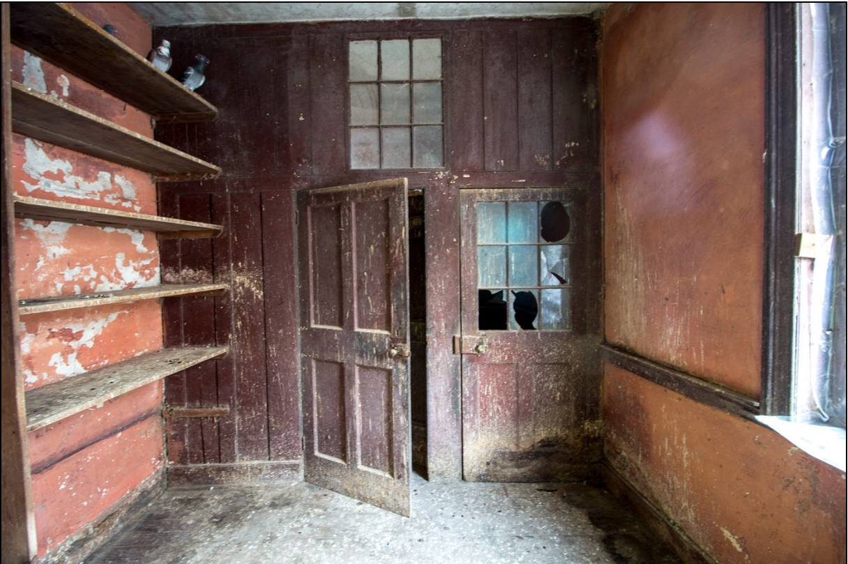
First floor room
