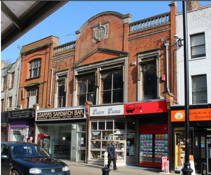
13-17 High Street – grant application approved for new shopfronts and brickwork repair
