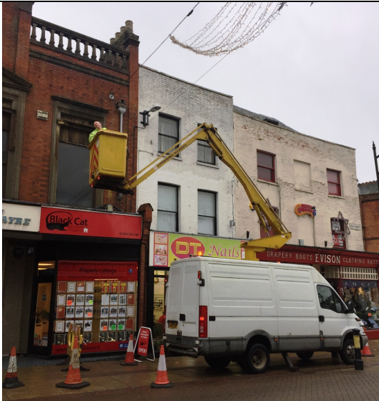
Gutter Cleaning on Wisbech High Street, November 2018
