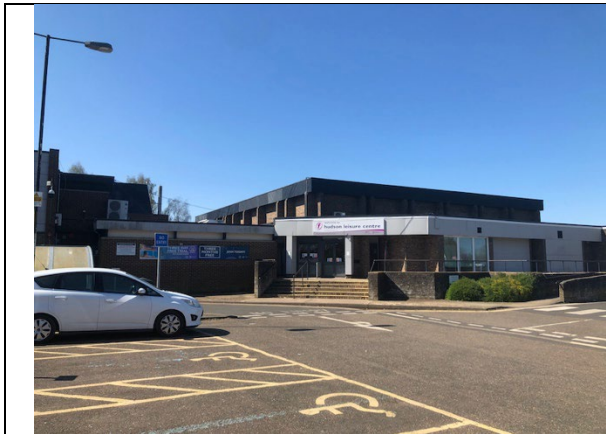
Exterior of building
