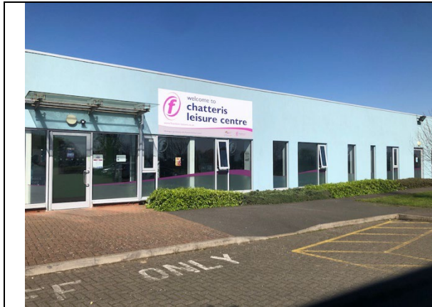
Exterior of building
