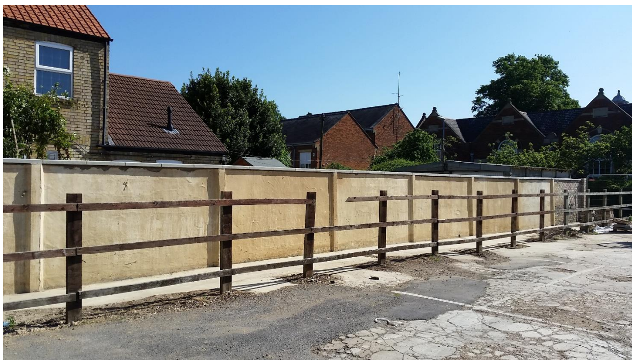
Completed Works Photo Darthill Road Car Park
