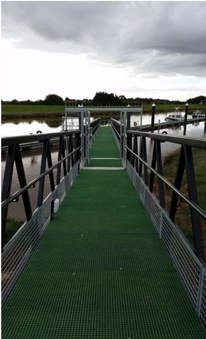
Progress Photo – Marina Access Brow and Pivoting Walkway
