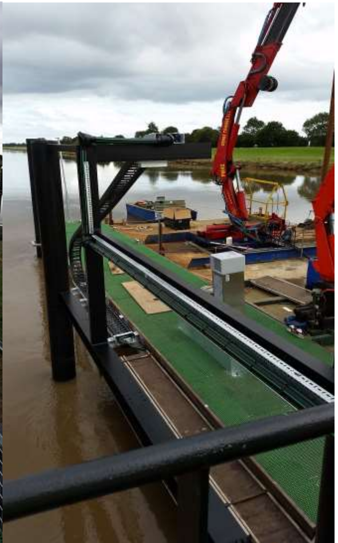
Progress Photo – Commercial Vessel Fuel Facility
