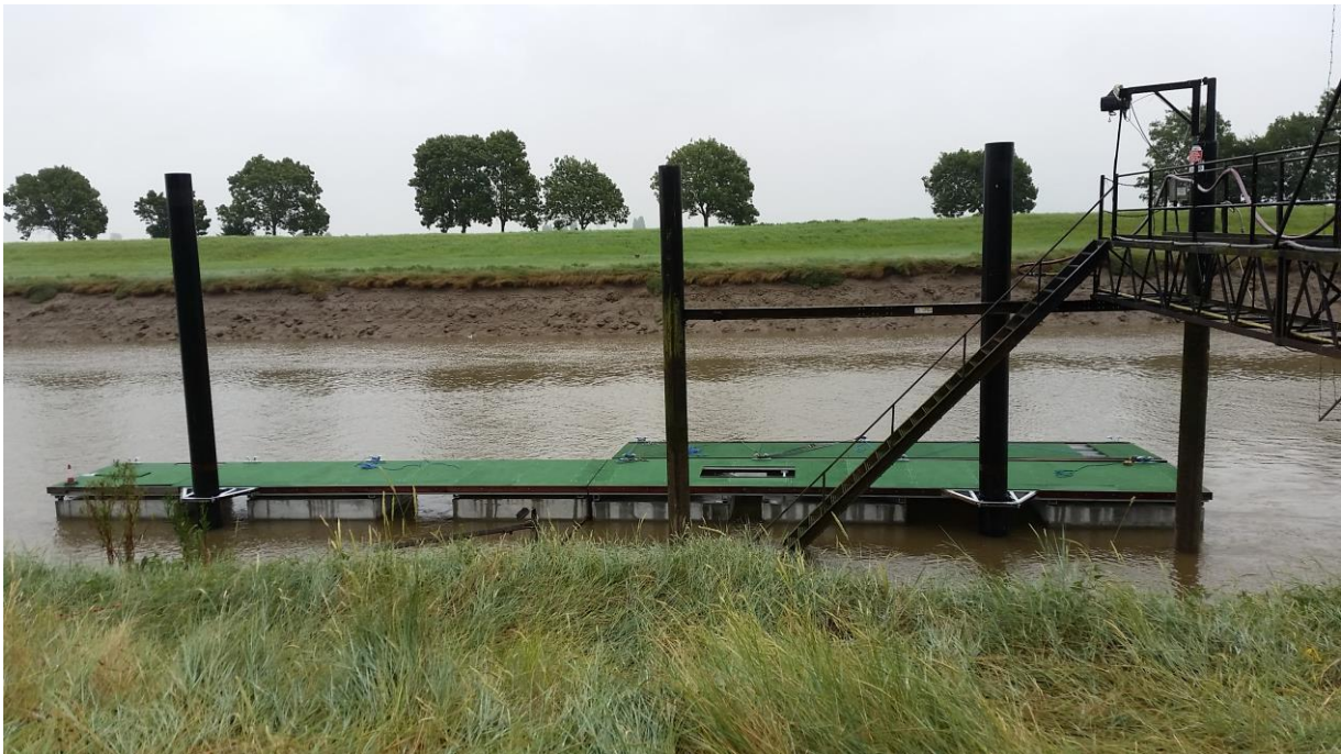
Progress Photo – Commercial Fuel Berth Facility Pontoon Erection
