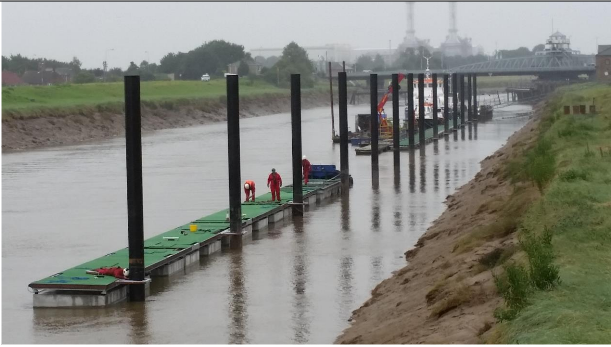
Progress Photo – Commercial Fuel Berth Facility Pontoon Erection
